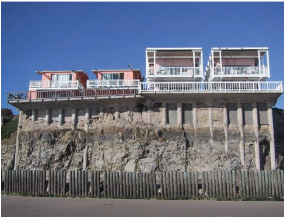
Ocean waves eroded the cliff base of these houses until the support columns were revealed.
