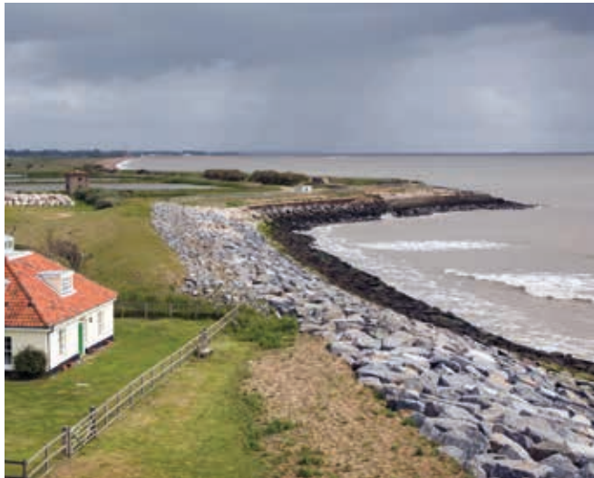
The hard surfaces of the large rocks mitigate the erosion of the land between the house and the water.
